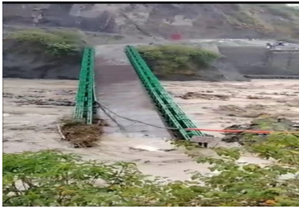
Fig. 1: Collapsed Bridge, Source: Google Source: Open access social media
