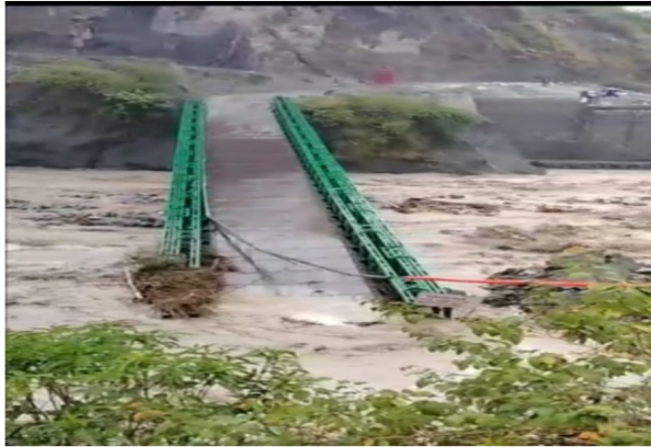
Fig. 1: Collapsed Bridge, Source: Google Source: Open access social media
